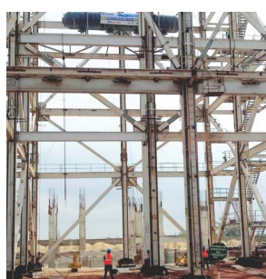
Boiler drum lifting of 125 MW Sendou Coal Fired Thermal Power Project, Senegal.
