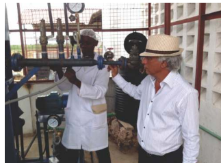
Instaaltion of boiler for juice plant
