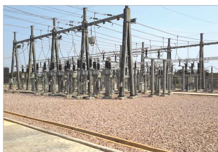
6633 KV Substation with Incoming & Outgoing Bay 3
