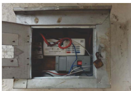
Meter Connection to House Hold
