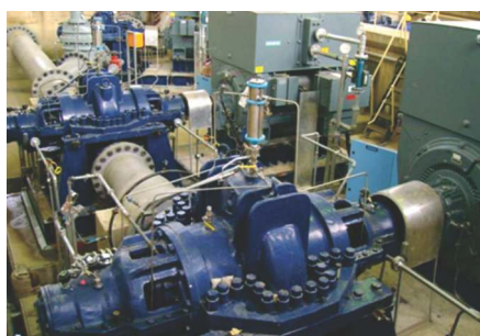
Kirloskar split-case pump sets installed at RAND WATER BOARD, SOUTH AFRICA, provides drinking water to GAUTENG Province
