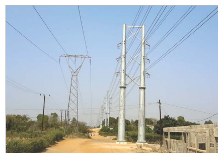
Double CKT 66 KV Transmission Line-1
