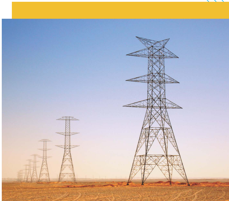
500 kV DC Triple Conductor Transmission Line, Egypt
