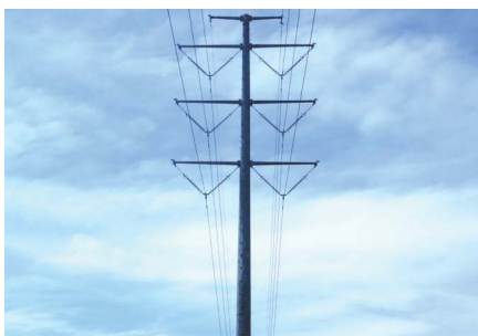
132 kV DC Monopole Transmission Line, Uganda
