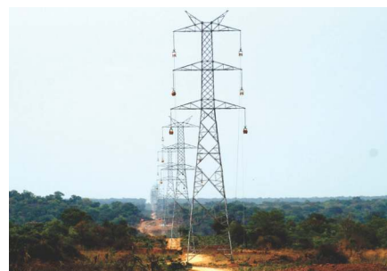
330 kV SC Transmission Line at Zambia
